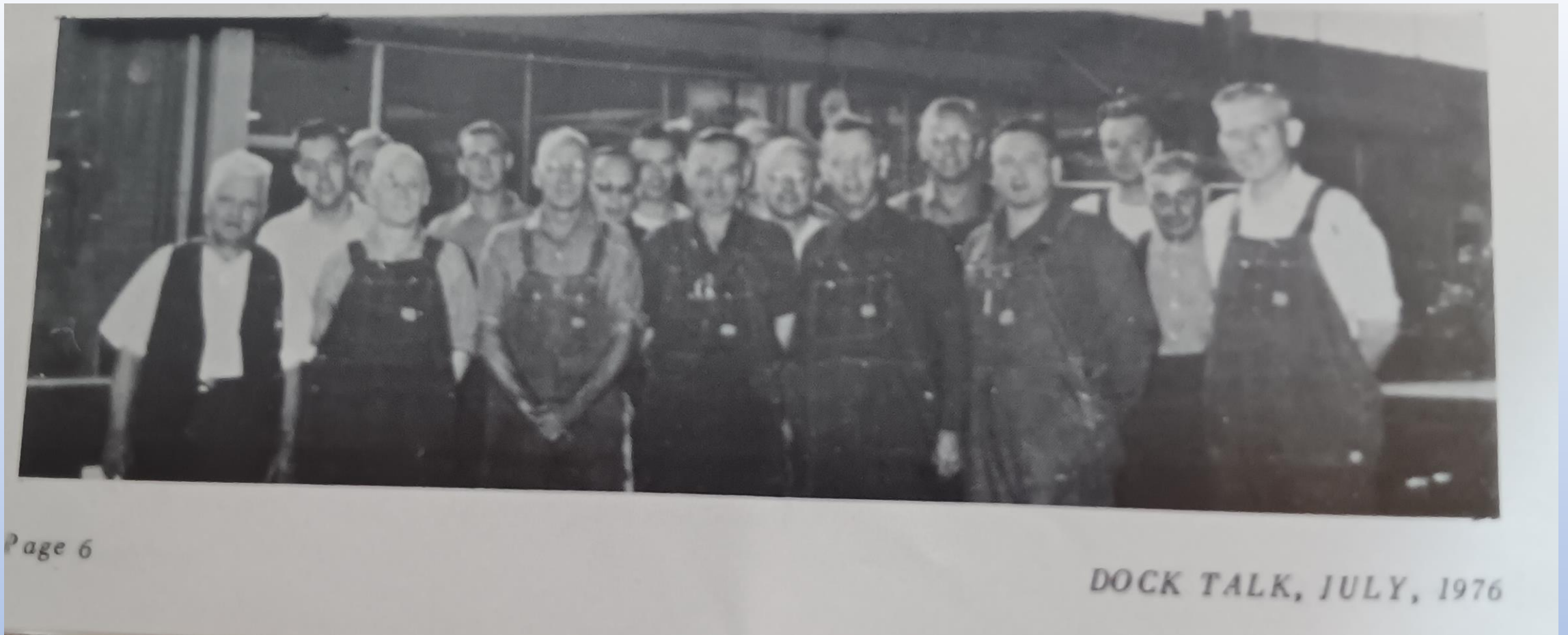
During the Pittsburgh & Conneaut Dock's first open house on July 28, 1951, The personnel of the machine shop gathered to make this portrait. Two people who are partially hidden are listed as unidentified. The Machine Shop members are left to right: Jake Koelliker, foreman; Pat Nimelli; unknown; Charles Hawley; Guy Vorse; Paul Hawley; Leon Webster; Bill Lyon; Francis Bryant; Unknown; Winfred Golden; Ray Smith; Herb S. Hopkins; Harold Beckwith; Bert Denkelberg; Clarence Bricker; and Bill Ahlberg.
