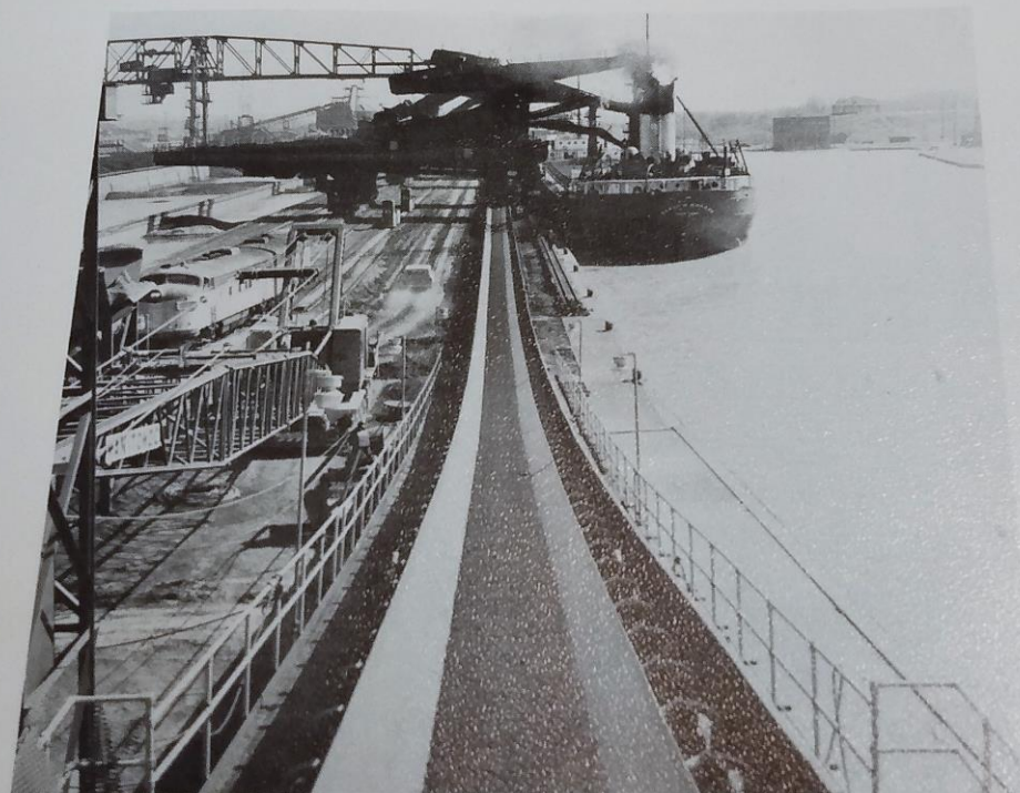
ORE DOCK VIEW WITH HULETT UNLOADERS TRANSFERRING IRON ORE PELLETS FROM LAKE FREIGHTER ONTO DOCK FRONT CONVEYOR BELT TO GROUND STORAGE. RATED CAPACITY OF FIVE UNLOADERS EXCESS OF 5,000 TONS PER HOUR
