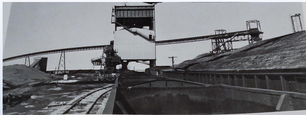
RE-LIMESTONE LOADOUT STATION, CAPABLE OF LOADING 400 100-TON CARS EVERY 12 HOURS. CARS MOVE BY RADIO-CONTROLLED LOCOMOTIVES AND LOADOUT CONTROLLED BY MINI-COMPUTER.
